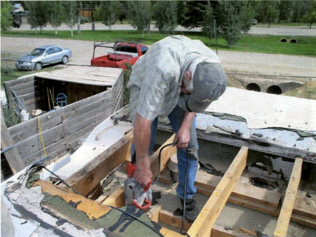
Above left – Ed Latham cuts through the roof rafters connecting the coach and addition. (Fortunately, these rafters did not penetrate the coach roof.) Above right – the side of the coach that had been covered for over 50 years by another interior wall in the addition is exposed. The floor joists in the addition are also now exposed and disconnected from the coach. Notice the “walk-through” opening cut into the side of the coach. This will eventually be closed again as part of the restoration project.
