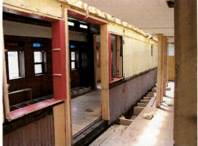
Above left – Ed Latham cuts through the roof rafters connecting the coach and addition. (Fortunately, these rafters did not penetrate the coach roof.) Above right – the side of the coach that had been covered for over 50 years by another interior wall in the addition is exposed. The floor joists in the addition are also now exposed and disconnected from the coach. Notice the “walk-through” opening cut into the side of the coach. This will eventually be closed again as part of the restoration project.
