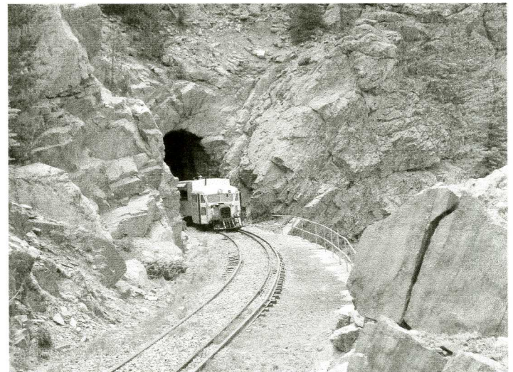
Exiting Toltec Tunnel (Rock Tunnel) (M.P. 315.2)
